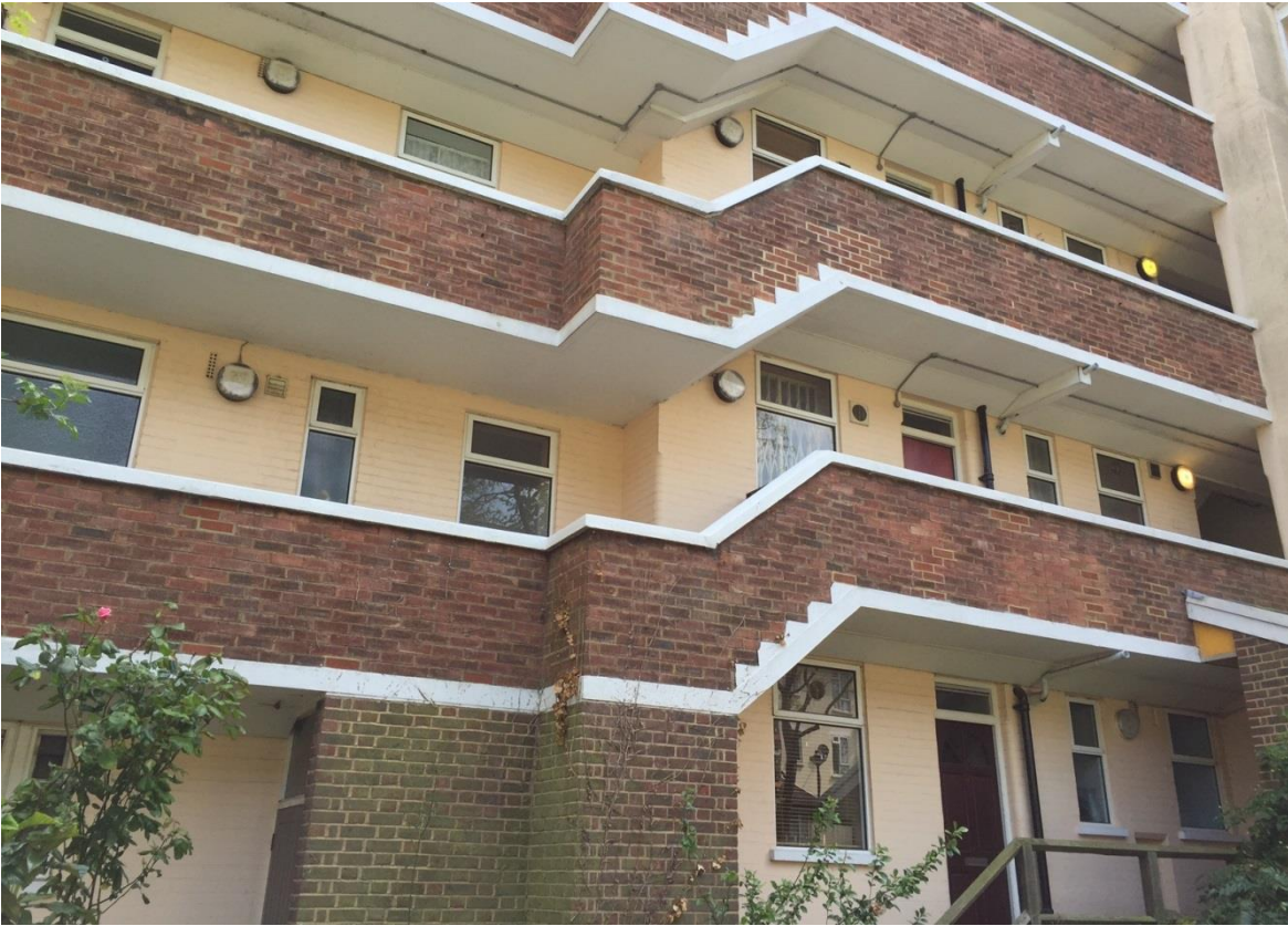
Image 4: North (courtyard) elevation of Mary McArthur House.
