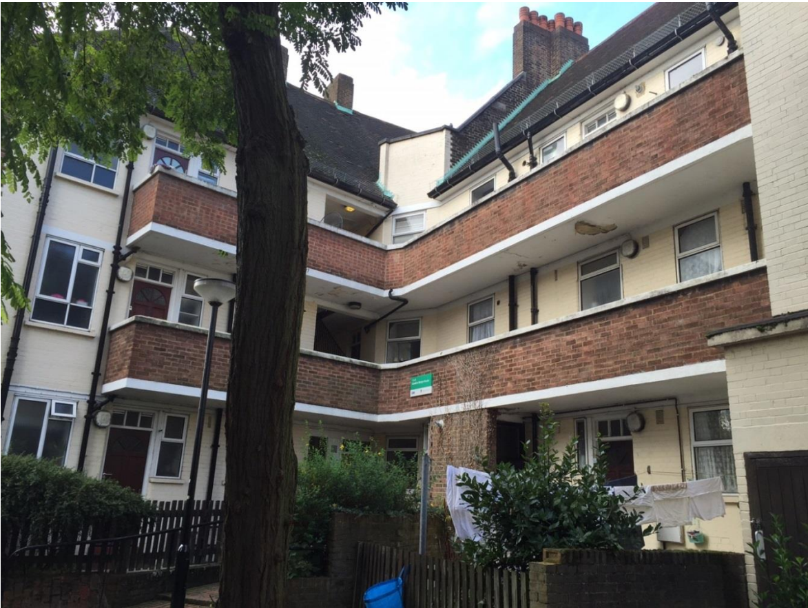
Image 5: South and East elevations of Caroline Martyn House.
